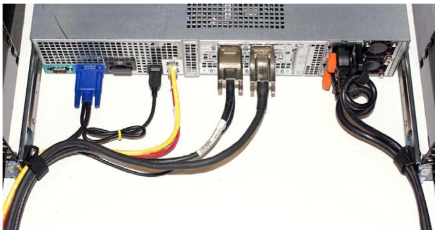
Figure 11: Cabling a System Installed in Static Rails
